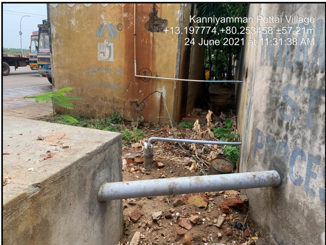
Bore well and Sump Supply
